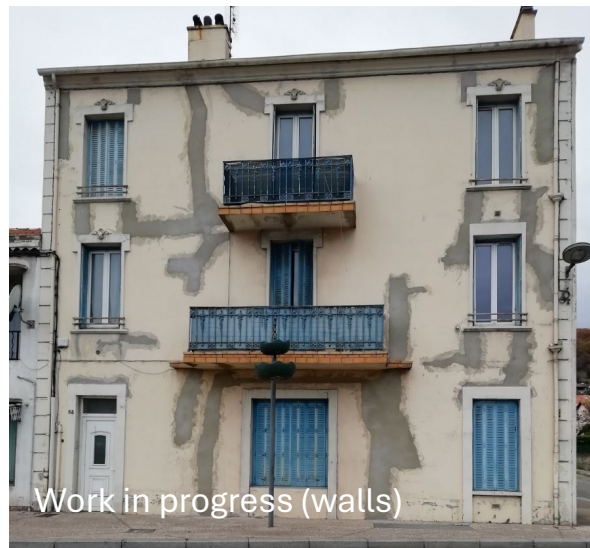
Reinforcement with tie rods
